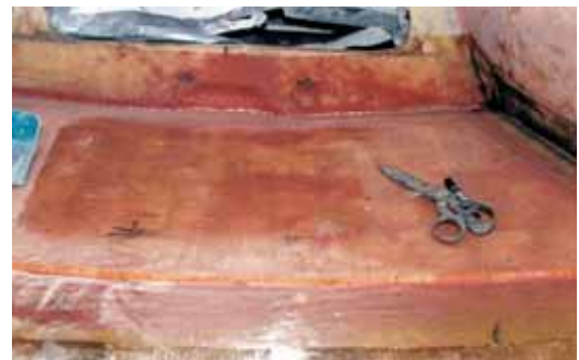
New balsa core and fiberglass skin were installed in the damaged areas.
